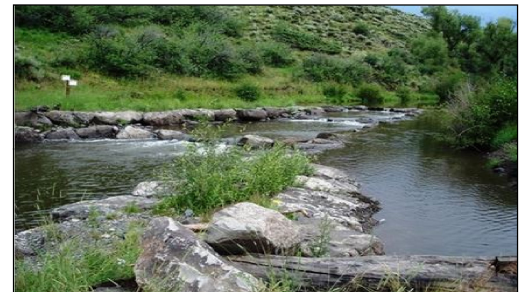
Rock Cross Vane with Diversion
