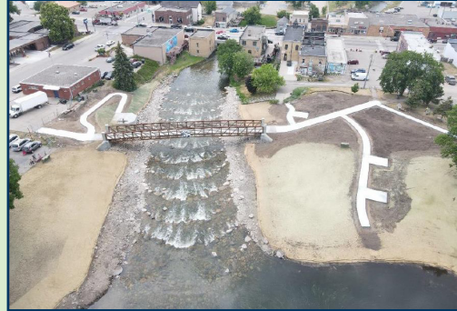
The deteriorating dam in Pelican Rapids was modified into a Rock Arch Rapids winter 2022/2023. The ramp gradually steps down the water 5 feet over 12 arches.
