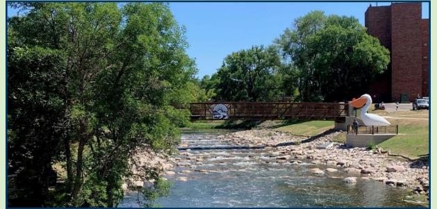
The deteriorating dam in Pelican Rapids was modified into a Rock Arch Rapids winter 2022/2023. The ramp gradually steps down the water 5 feet over 12 arches.
